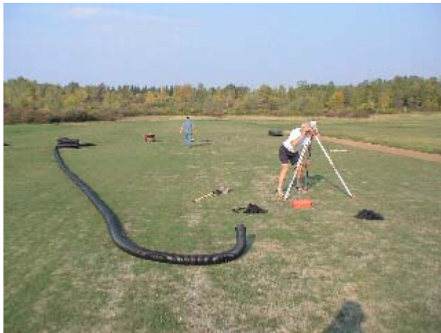
Getting the slope right takes real skill
